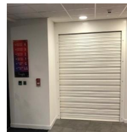
Tubular motor fire shutter Manchester University
